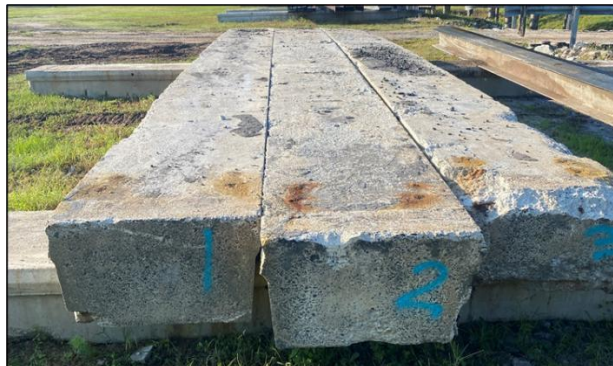
(a) Beams in contractors' yard
