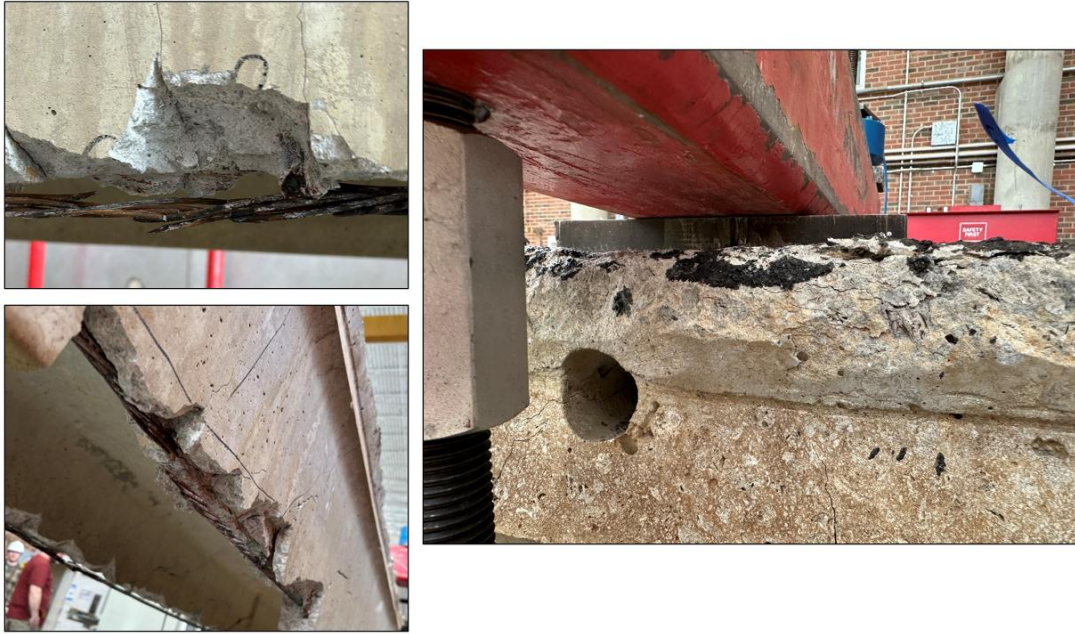
Figure 4-4: Specimen WCU1 at failure
