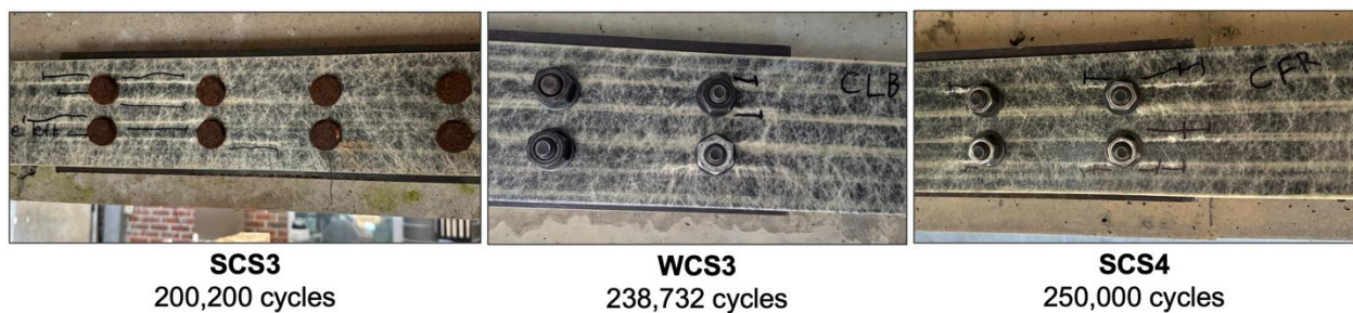
Figure 5-5: Condition of FRP straps at the conclusion of fatigue cycles
