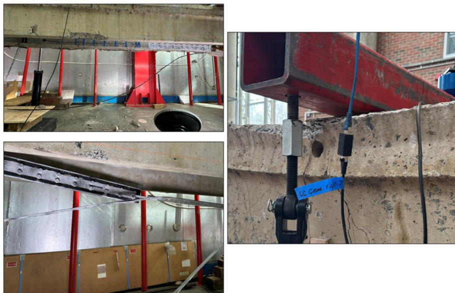
Figure 4-5: Images of SCS1 at failure
