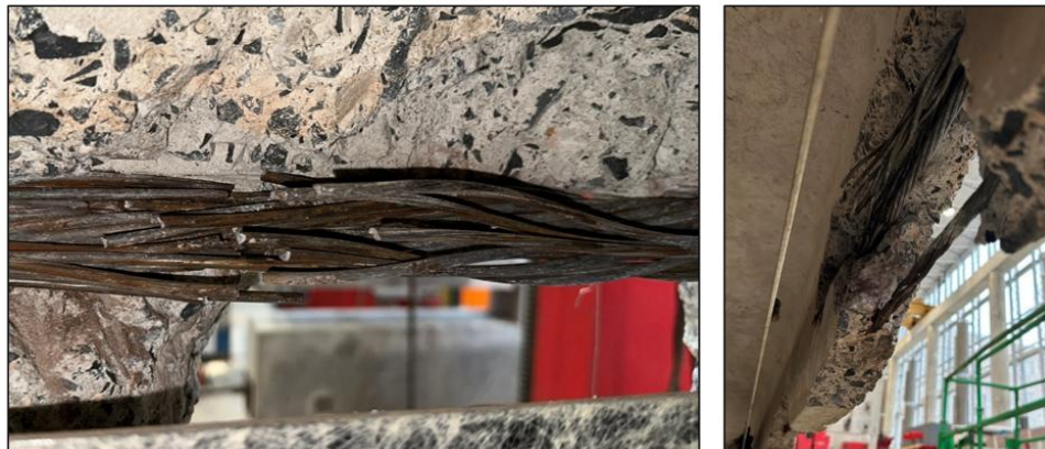
Figure 4-19: SCS3 at the end of fatigue testing.
