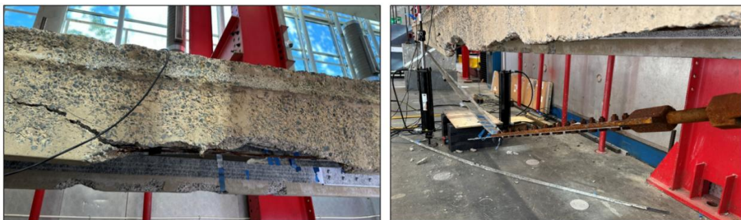
Figure 4-7: Specimen SCS2 at failure
