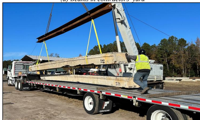
(b) Loading of beams onto truck
