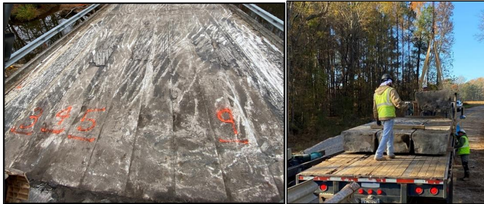
(a) Beams prior to removal
